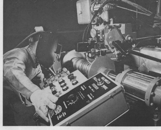
CIRCUMFERENTIAL AUTOMATIC welding machine is operated by Charlie Bates. The welding head, controlled electronically, moves up or down to hold the welding quality uniform.
